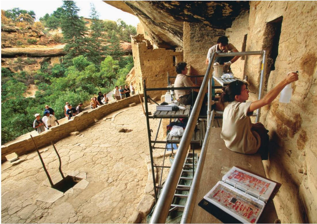
Anthropological archaeologists from the University of Pennsylvania work to stabilize the original plaster at an Anasazi (Native American) site in Colorado's Mesa Verde National Park. © George H.H. Huey/Alamy Stock Photo
